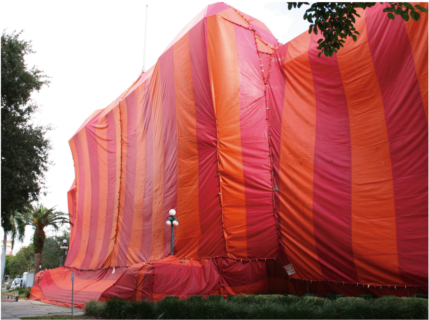
Figure 13. During structural fumigations, gas must be released into the structure and held for a specified period. The gas is confined either with a tarp or by using tape to seal all areas where gas might be able to escape.
