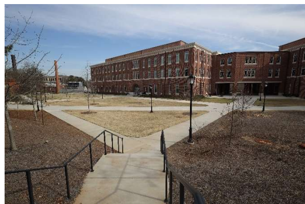
Figure 21: View from the south stair entrance.
