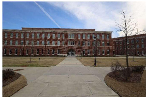
Figure 20: View of I-STEM Building I
