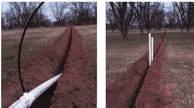
Figure 4. Installing PVC mainline.
