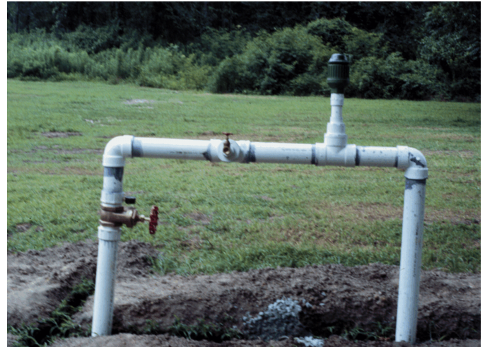
Figure 8. Control station with manual on-off valve (left valve), injection port (center valve) and kinetic air relief valve (right valve).
