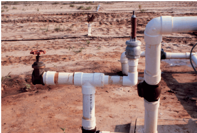
Figure 7. Control station with flush valve (left) and pressure relief valve (right).
