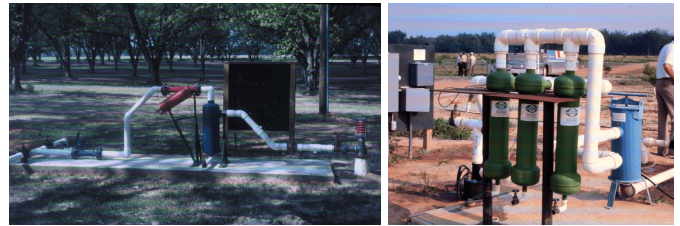
Figure 19. Screen filter and vortex sand separator installations.
