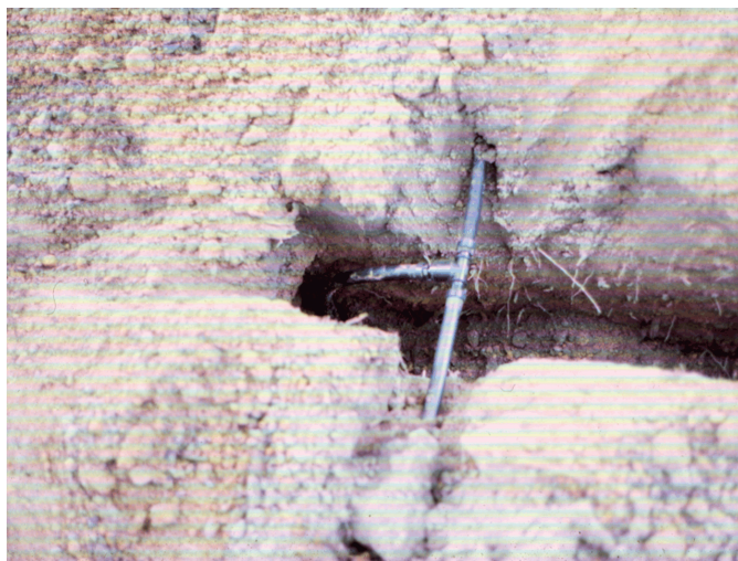
Figure 16. Connecting lateral line to PVC.
