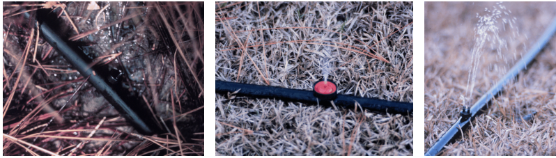
Figure 10. Above ground installation of emitter and lateral line.
