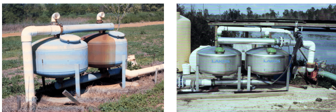
Figure 18. Sand (media) filter installation.
