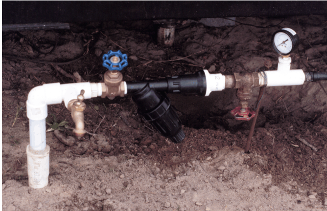
Figure 6. Control station with (from left) manual on-off valve, filter, pressure regulator, secondary manual on/off valve and pressure gauge.
