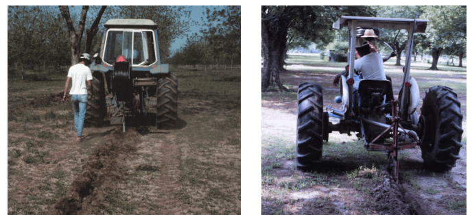
Figure 14. Installing lateral line using subsoil plow. Rear mounted equipment (left) and both front and rear mounted equipment (right).
