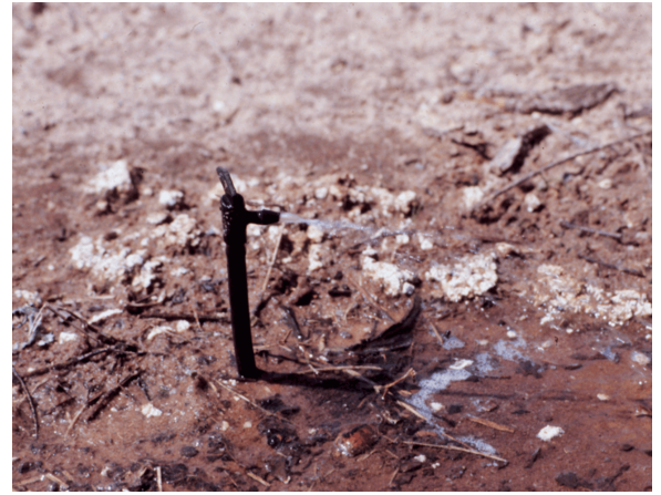
Figure 12. Below ground installation of lateral line and above ground installation of emitter.
