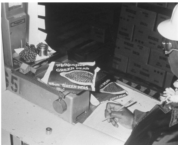
Figure 7. In-line check weight of packaged product.
