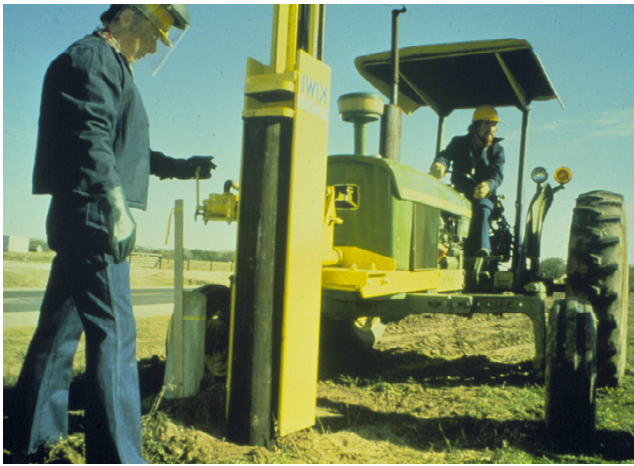
Figure 11. A tractor-mounted post driver.
