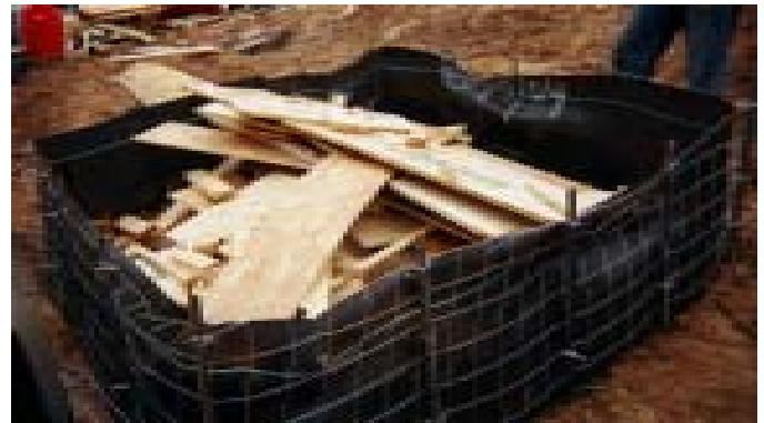
Example of a wood waste storage area.
