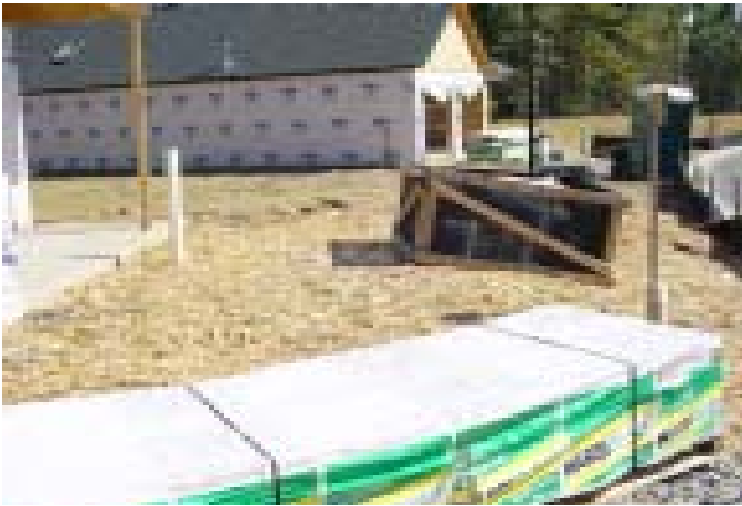
Ground wood waste used for a delivery pad.
