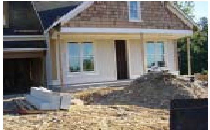
An example of ground wood waste at the construction site
