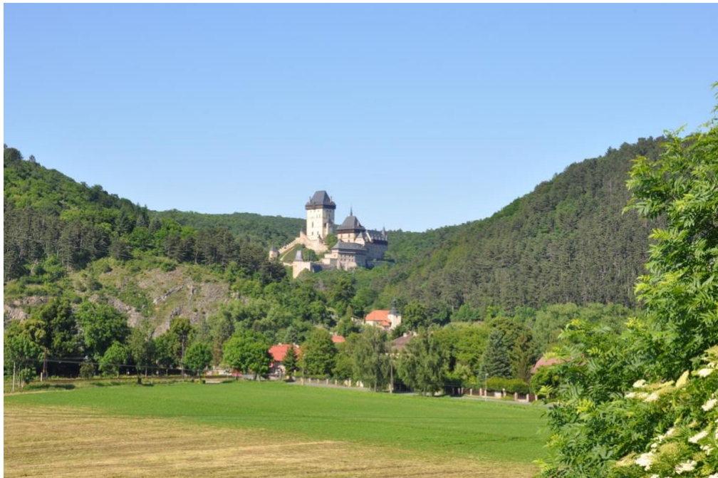
Figure. 11 View of the Vista Surrounding Karlstein , Karlstein, Czechia, 1348-1372. Image source: https://www.hrad-karlstejn.cz/en/photogalleries/43104-exterior
