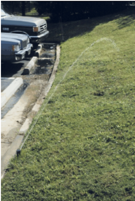
Figure 10. Low pressure on a sprinkler creates “donut” shaped patterns because droplets do not break up.
