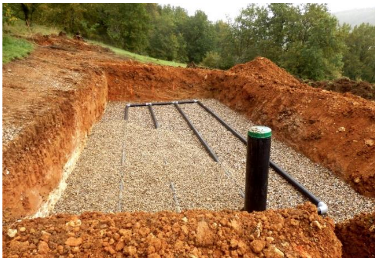
Figure 5: Sand Filter Under Construction. (EPA 2021).
