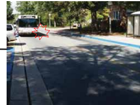
3 DRAINAGE GRATE & GUTTER CREATE A HAZARD FOR CYCLISTS. BIKES & VEHICLES OFTEN PASS BUSES AT STOPS
