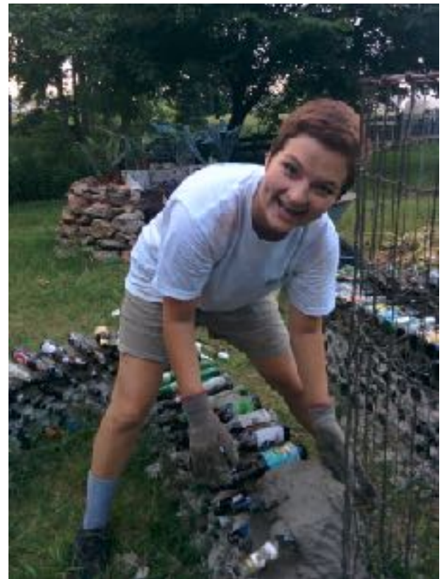
Putting in the layer of wet concrete to anchor the bottles (and having a bit of fun while doing it!)
