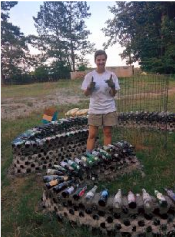
Sarah Bess Jones finishing up the second phase of building the bottle and concrete keyhole Campus Sustainability Grants Program (2013-2014) REV 08.26.13
