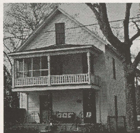
Folk Victorian building style, Side Hall building type
