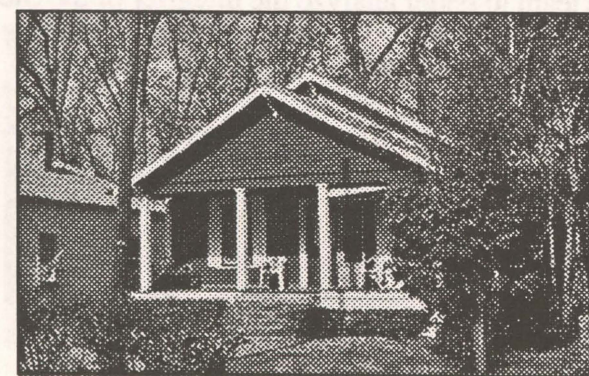
Bungalow building type, Oak Street
