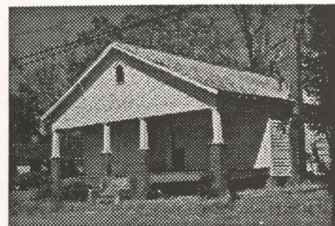
Vacant Bungalow in good condition
