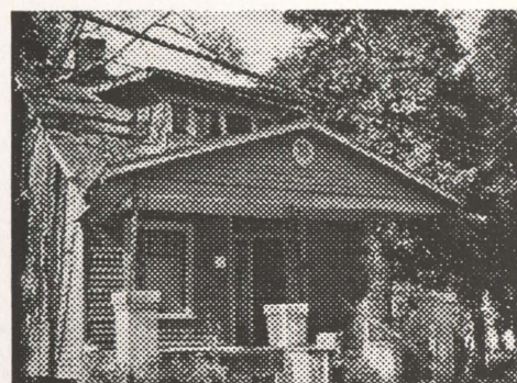
Vacant Bungalow, in derelict condition
