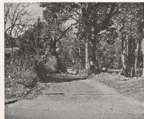
Unpaved section of Small Street, Thomasville
