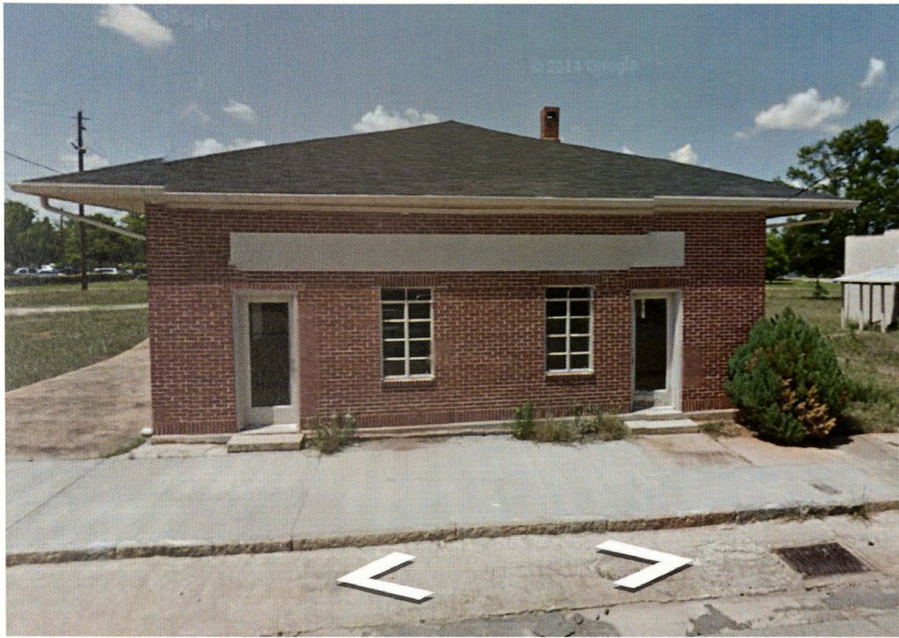
Two buildings exist on site, formerly affiliated with the Sandersville Railroad Depot.
