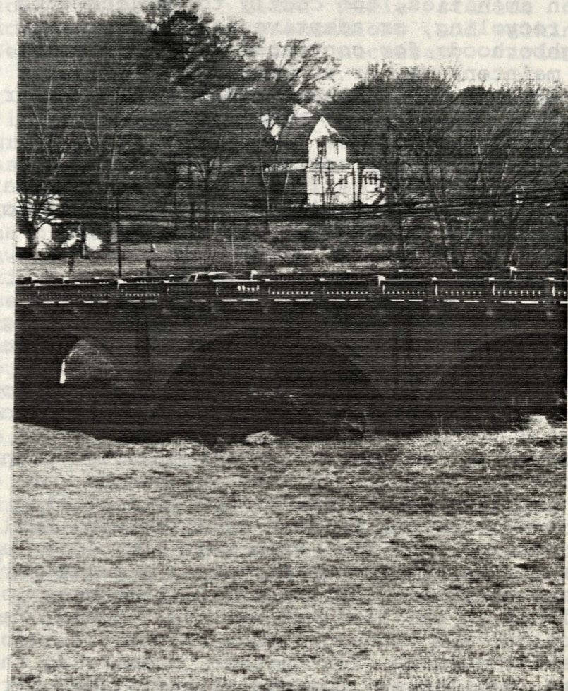
Southeast view across Curry Creek Bridge
