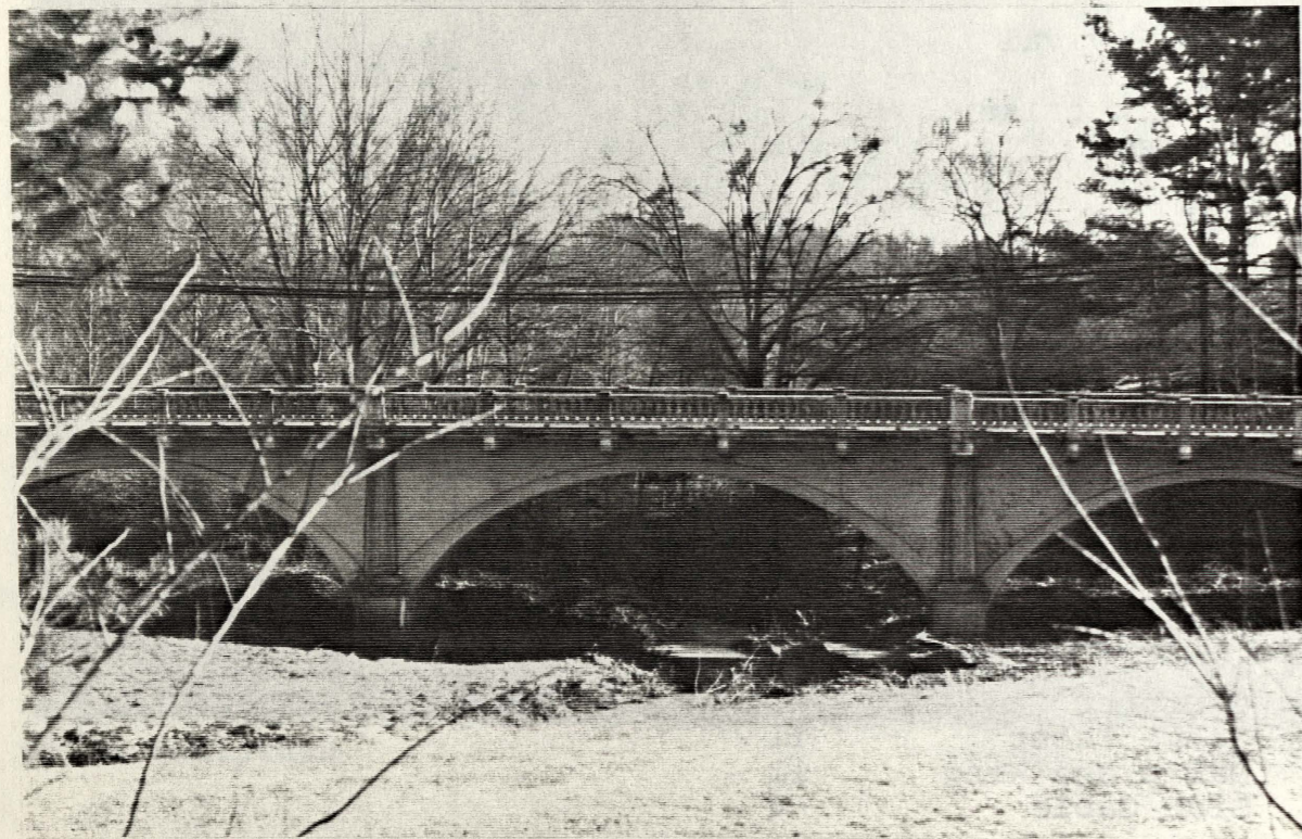
Solid Spandrel Concrete Arched Bridge
