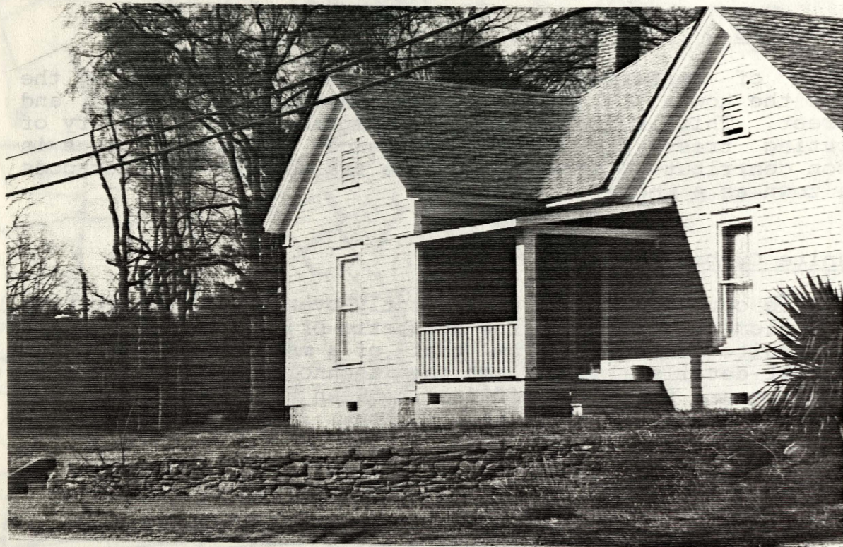
Rubble Masonry Retaining Wall
