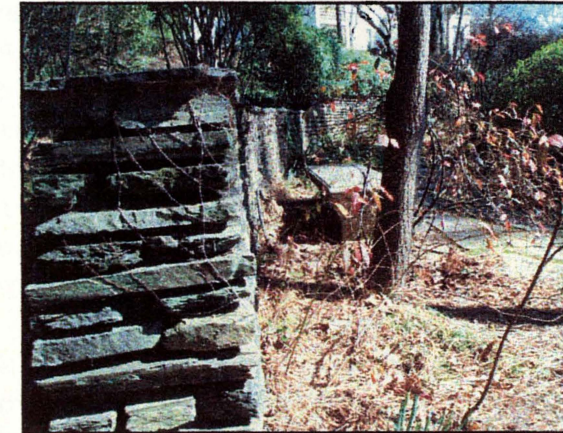
Figure 34. Stacked Slate retaining wall
