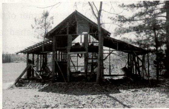
Fig. 5 – Barn at southwest corner of property; all siding has been removed.
