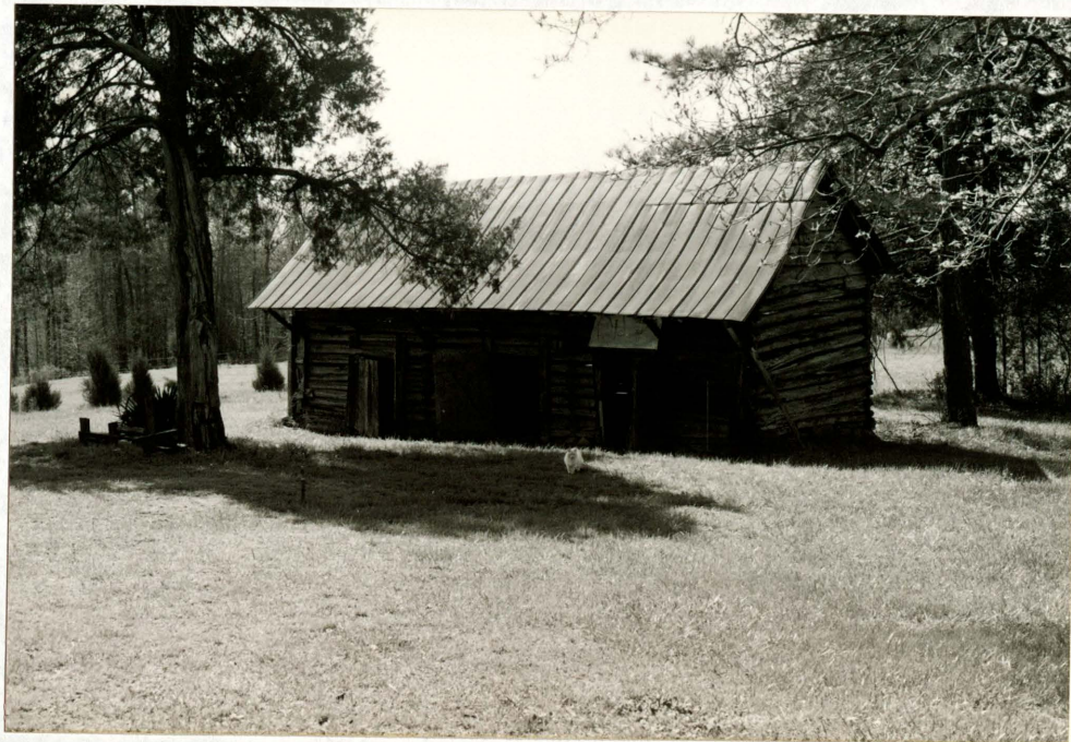
The log structure, now empty and about to be demolished.
