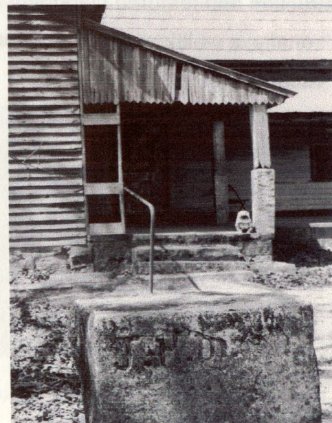
Fig. 1 – Initials “J.H.M.” on pier flanking the walk.
