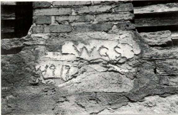
Fig. 2 – Initials and date etched in base of chimney, south elevation.
