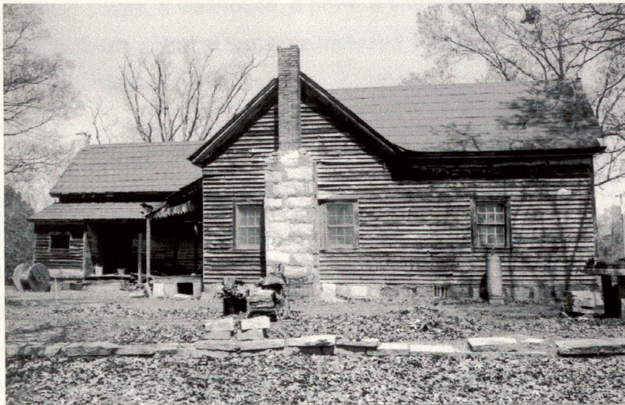
View of the cottage from the west, showing pressed metal roof, original windows and siding.
