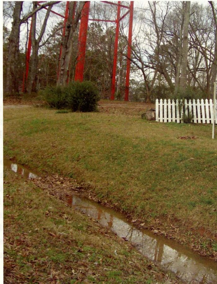
Swale draining overflow from water tower
