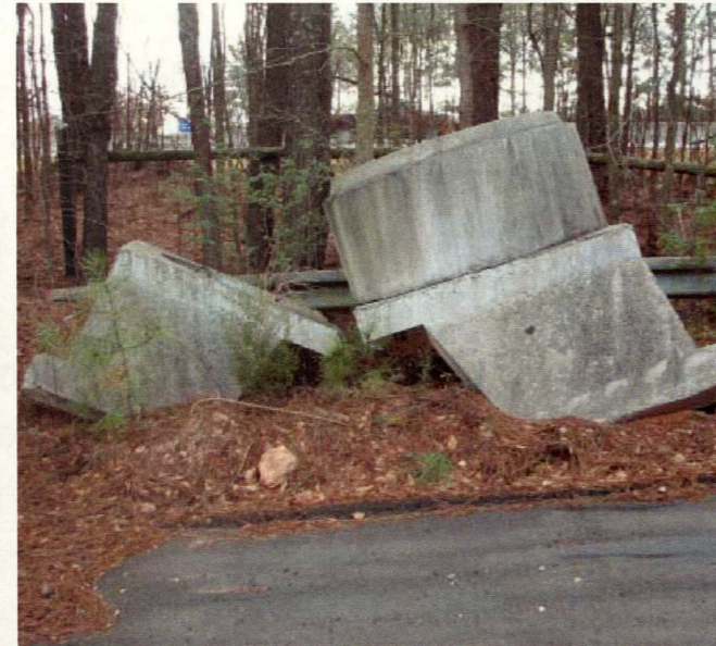
Stubbed out sewage vents and refuse public infrastructure material and equipment
