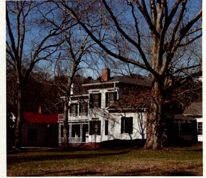
Mature trees and historic architecture
