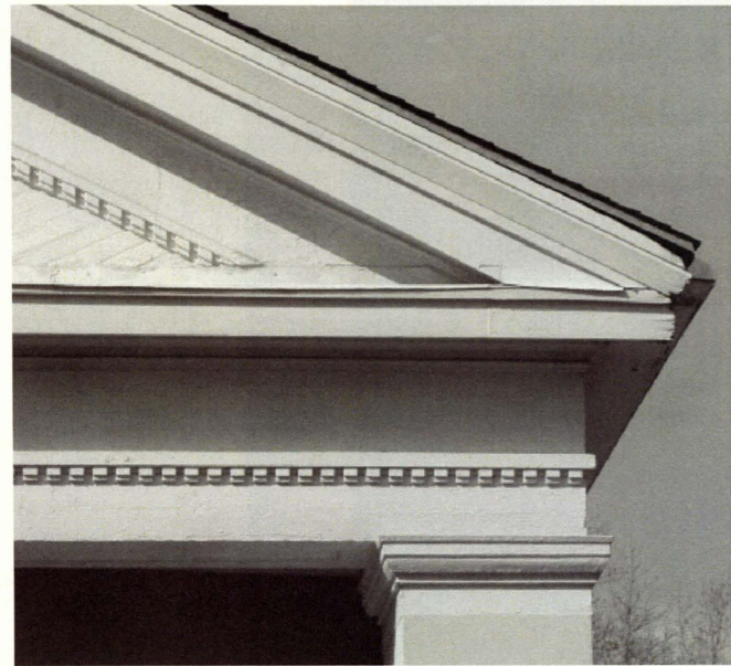
Historic buildings inside and outside the National Register Historic District
