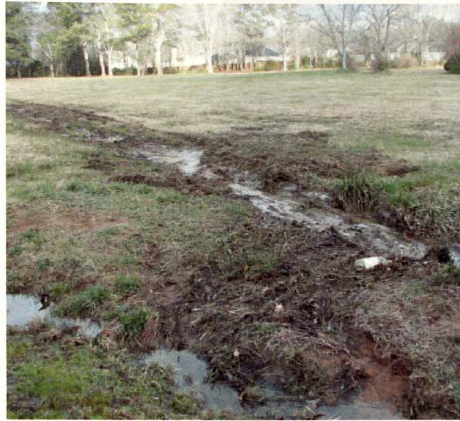
Standing water as well as overflowing water from the water tower
