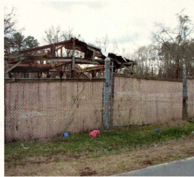
Maintenance shed area
