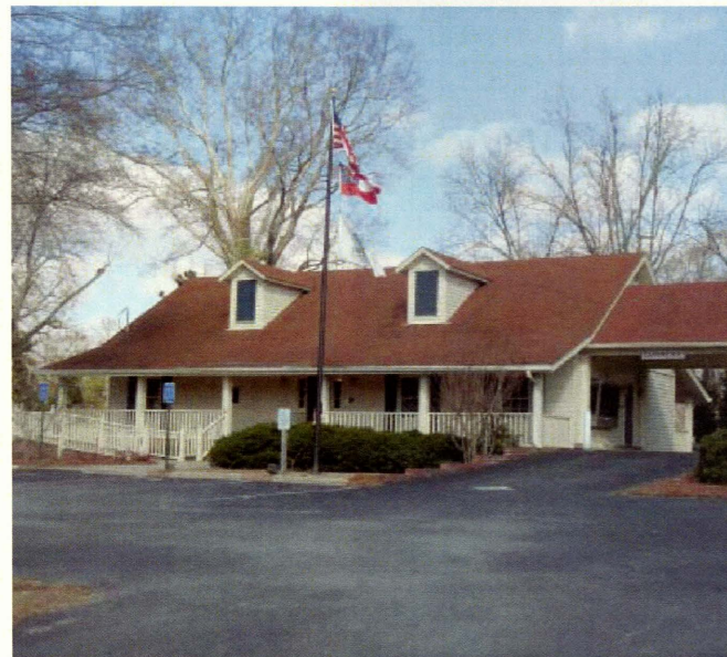
Town Hall is residential in design but does not reflect Oxford residential character
