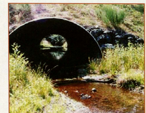
Example of a proper culvert system
