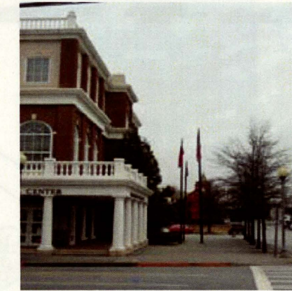
View from Courthouse to Historic Jail Building
