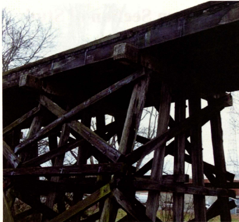
View of the railroad crossing
