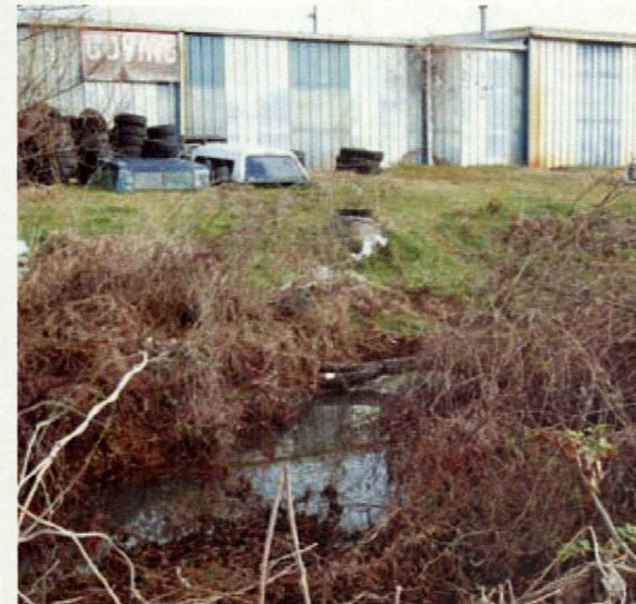
Impervious surfaces encroach on the creek
