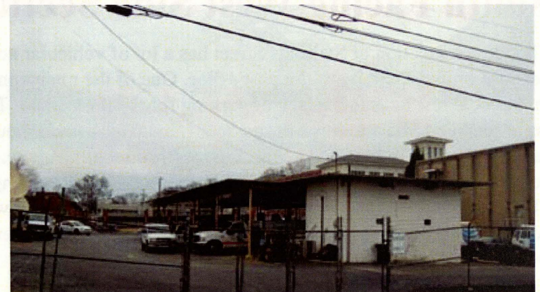
Parking lot used by AT&T for service vehicles
