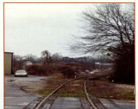
Abandoned rail system
