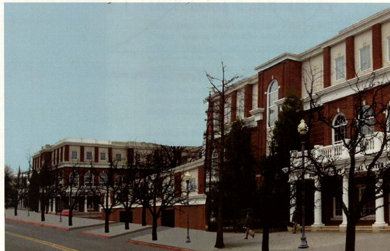
After: Judicial Center is linked to future expansion of government facility by a two story secure parking garage for both public and secure use. Sidewalk improvements will increase mobility throughout site
