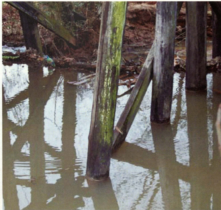
View of the railroad crossing
