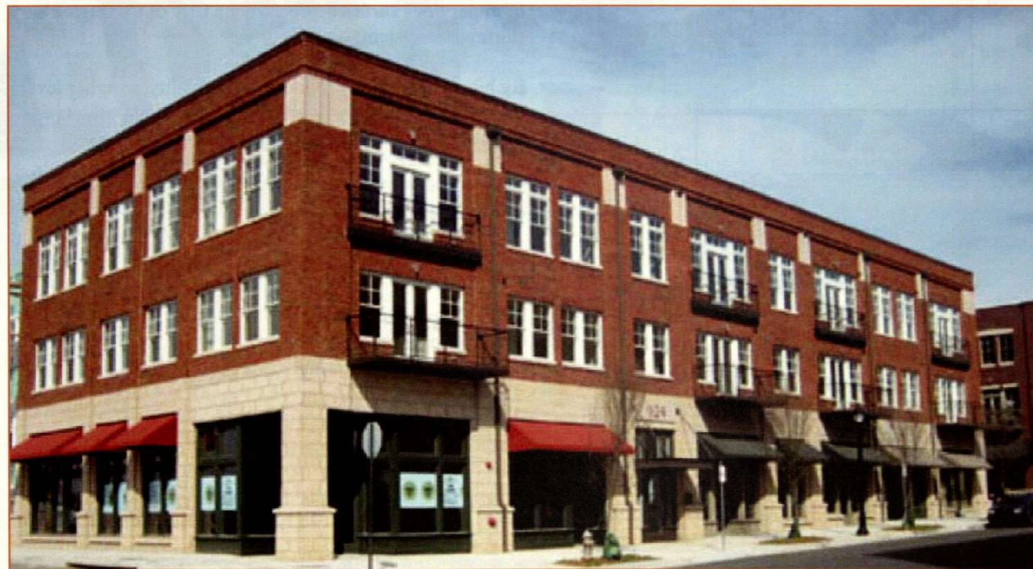
Commercial building in Glenwood Park
