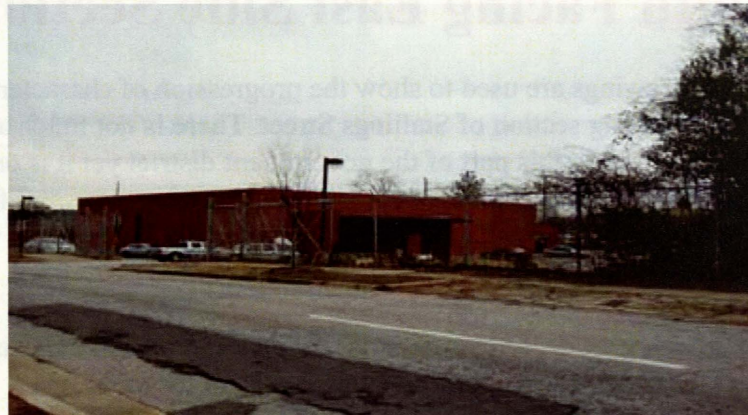
The view of the Post Office from Lee Street
