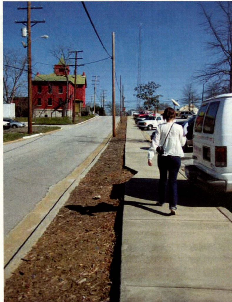
Before: Stallings Street facing North-East. Sidewalks are only available on one side of the street and there is no aesthetic character
