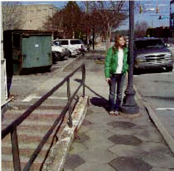
This portion of the sidewalk is too crowded and allows a mere two feet for pedestrian passage, which is inadequate to accommodate wheelchairs.
