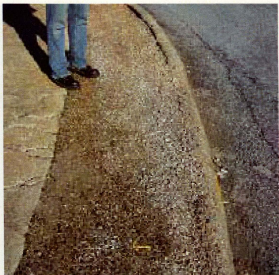
Another sidewalk and buffer in disrepair with a shallow and broken roadside curb.
