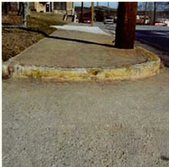
This curb cut is not ADA accessible.
