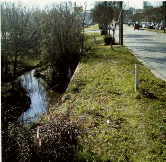
Stormwater runoff is poorly managed and the proximity of the retaining wall is a hazard for pedestrians. Absence of a sidewalk has caused worn out grass strips.
