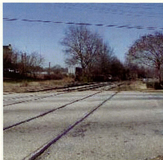
The railroad break in the sidewalk creates a challenge to pedestrians because of the unlevel surfaces.
