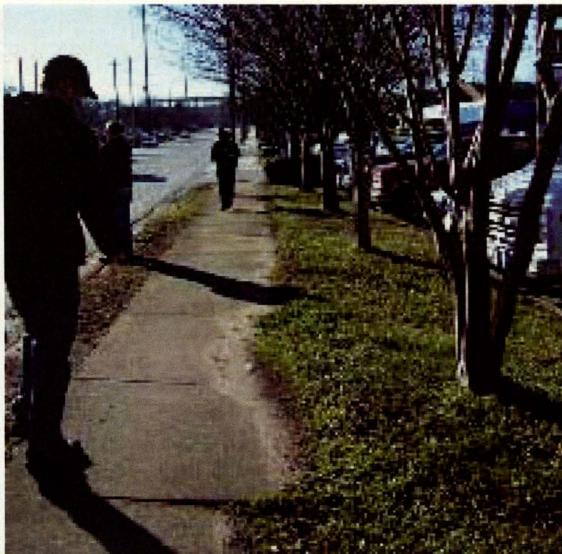
Unkempt buffers have grown over the walkways in some areas degrading the quality of the sidewalk for pedestrians.
