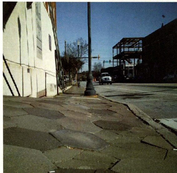
Many of the walkways are uneven, causing hazards for the crossing pedestrians.
