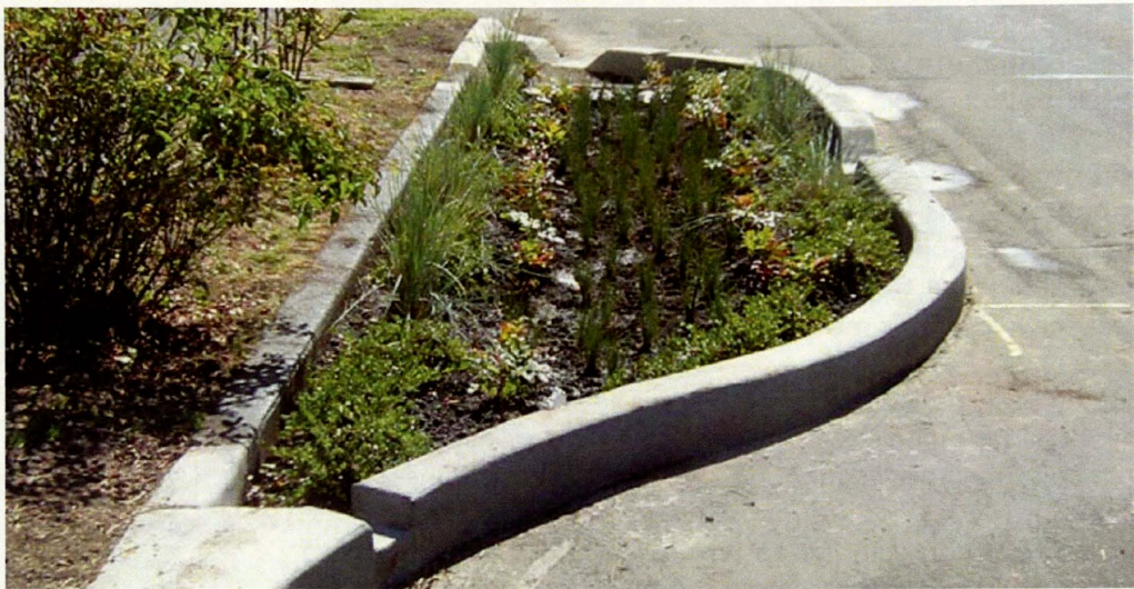
Typical curb alternatives that could be used throughout the Pace Street Corridor. Stormwater runoff enters through the intakes at the rear and sides, infiltrates to a certain capacity, and exists through the curb overflow at the foreground. (SE 57th Avenue & Ankeny Street, Portland, Oregon. Photo courtesy: City of Portland Bureau of Environmental Services Stormwater Management Manual)
