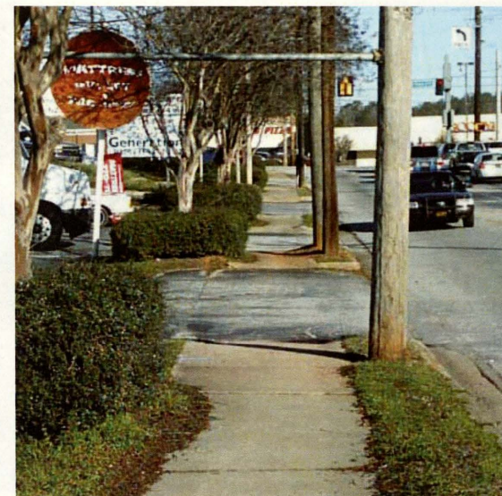
Telephone poles with horizontal extension lines creates an obstruction to pedestrians, located a mere 2.5' above an average man's height.
