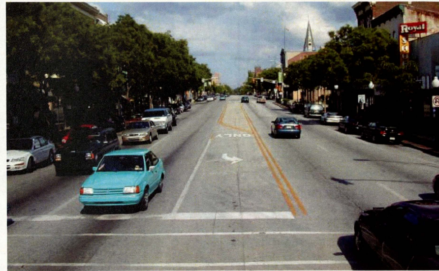
Typical urban street shown before road diet. Existing conditions show a roadway with four travel lanes, a two-way turn lane, and parallel parking on both sides of the street.
