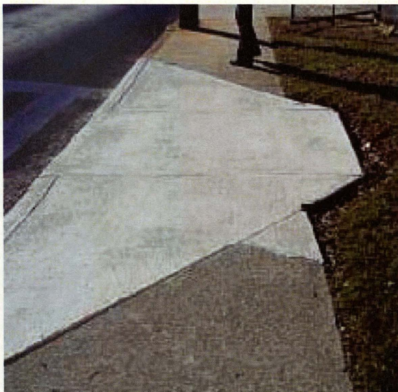
This handicap accessible ramp (located at a mid-block crosswalk) appears to go nowhere.
