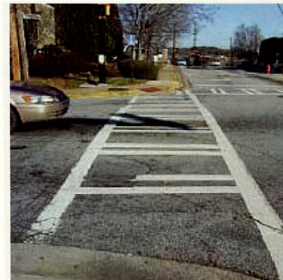
This crosswalk at the Usher Street intersection suffers from lack of maintenance, providing a struggle for pedestrians with strollers and citizens with wheelchairs.
