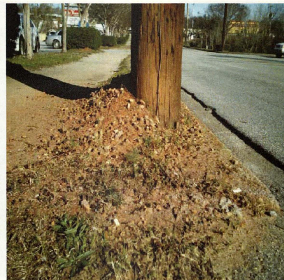
Grass strips have become severely eroded causing muddy streams from the drainage.
