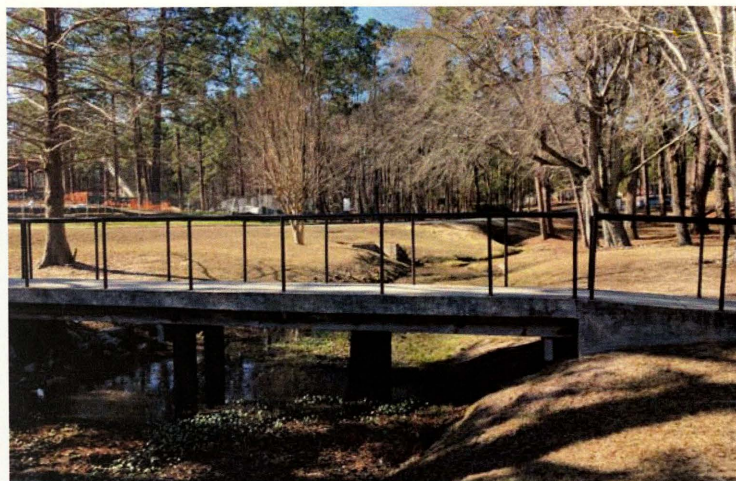
Bridge across Ezra Pond.
