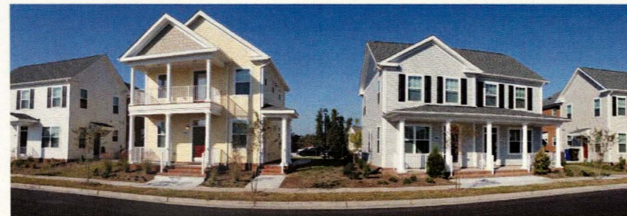
The building envelopes are air tight and efficient, and continuous insulation to the exterior Energy Star® windows help minimize heat gain/loss.
