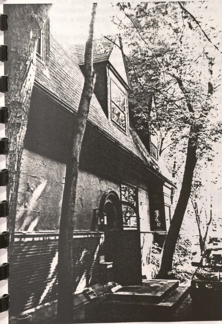
Beautiful entry on south side and sun-capturing bay windows. "Weed trees" are causing destruction to building and are not needed in this already shady location.
