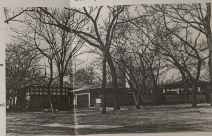
Mr. Pfeiffer's text from Monograph 3 (1988) could not be further from the facts observed on a personal field investigation. He wrote, "...it is sad, to say the least, to see this once great entity so split and cut into segments." It is unfortunate that all writers do not see for themselves the excellent and clever division of the property into five separate ownerships, accomplished in the 1950s. This division was possible, of course, only because of the original zone planning by Wright. Only the raised garden has been destroyed, but the new house added at this corner sensitively fits the overall scheme, and the trellis-pergola screens the structure and serves as a background for the sunken garden redesigned by the Howletts. No sense of splitting and separation into segments is found here, as happened at many other Wright properties, most disturbingly at the D. D. Martin Estate in Buffalo.
