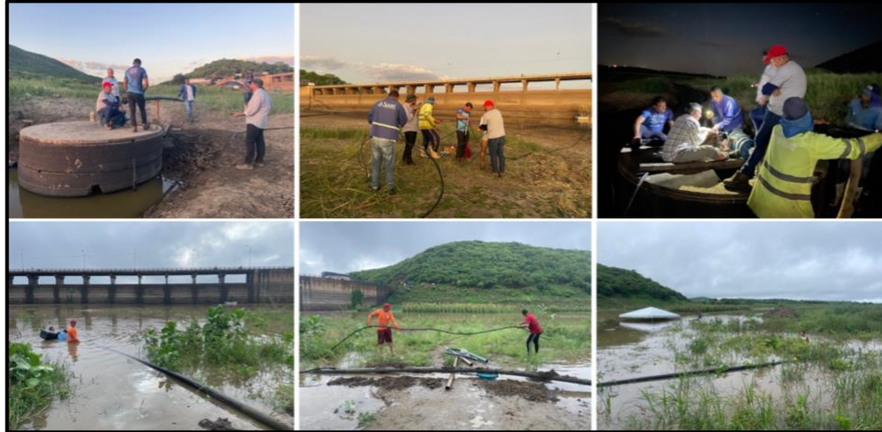
Figure 5.1 Preparing the Quixeramobim Reservoir for Water Supply Transitions.
