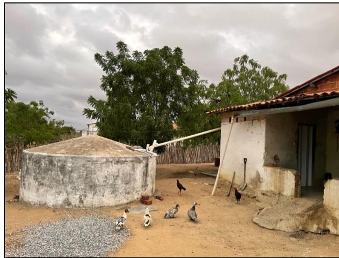
Figure 4.6 A household rain-harvesting cistern in the rural area of Quixeramobim, Ceará, Brazil, November 6, 2021. (Source: Author)
