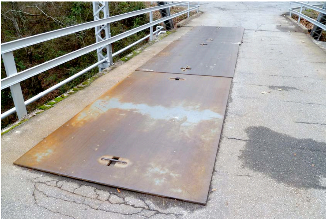
Fig. 6.3. Steel plates provided by the city for bridge repair. Photo by author
