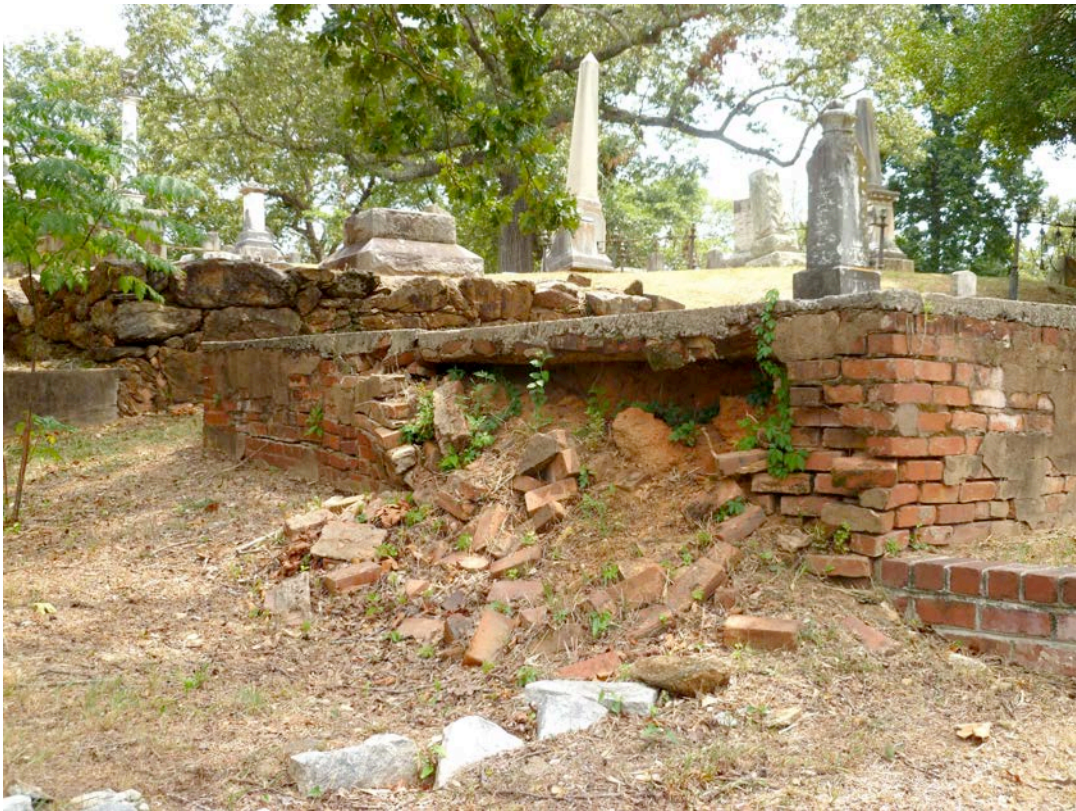
Fig. 4.2. Damaged retaining wall on West Hill. Photo by Author
