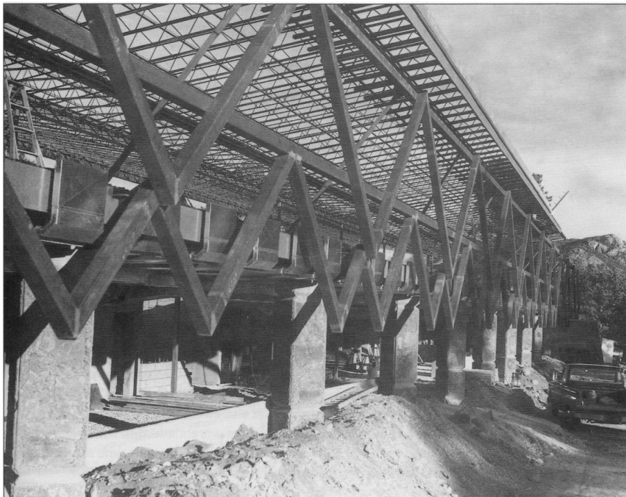
Figure 5.5. Exposed Cor-ten steel frame structure, 1966. 167
