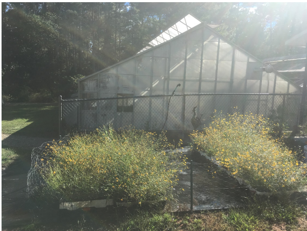
Figure 8. Photo of Block 1 (Mimsie Lanier Center) During Early August
