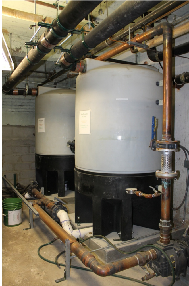
Figure 6.5: Water retention system in the basement 117
