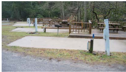
Figure 4.11 – RV parking pads with electricity
