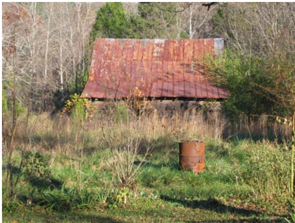
Photo 13—View east to the cow barn.
