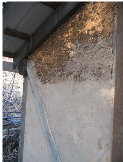
Slipstraw wall being plastered.
