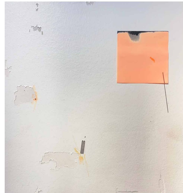
Thomas Street Flex Space wall during install – Photo by Ashley Wingo
