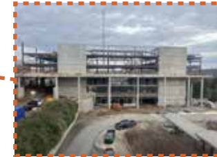
Arena (in-construction), in front of the Multi-modal Center
