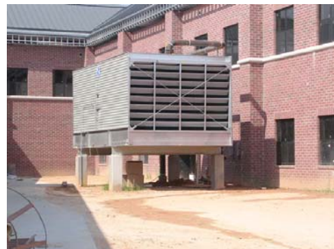
Figure 84. HVAC Water Cooling Tower
