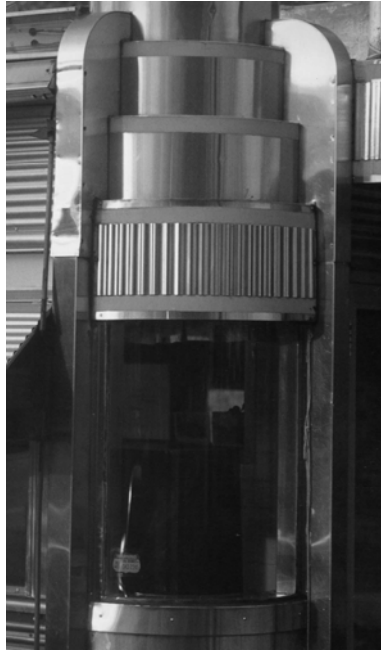
Figure 2-16. Fluted porcelain on a curved corner
