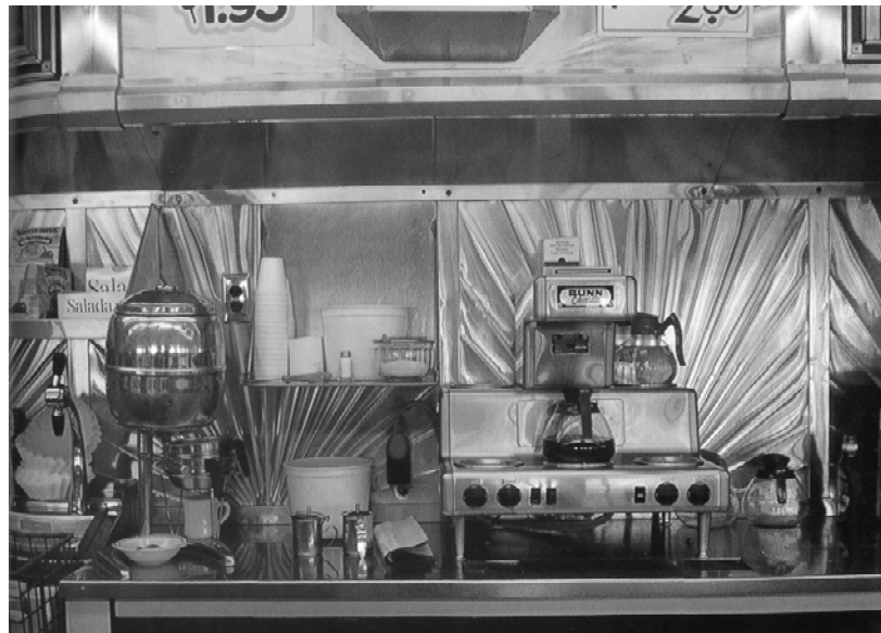
Figure 2-12. Stainless steel backsplash (Photo Courtesy of Robert O. Williams)
