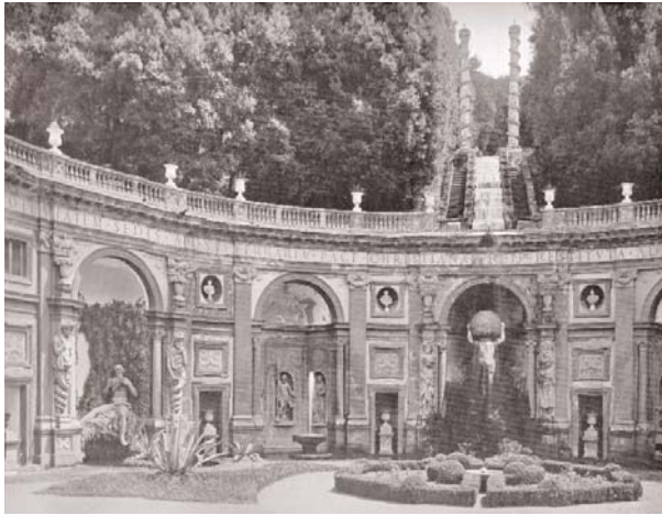
Fig. 4-18: Villa Aldobrandini, Water theater, Frascati (Bolton 1919, 174)
