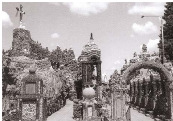
Fig. 6-44: Grotto of the Redemption, South wall, West Bend, Iowa (Brackman and Dwigans 1999, 66)
