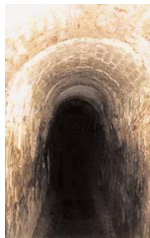
Fig. 7-16: Hellfire Caves interior passage (Walsh 1999)
