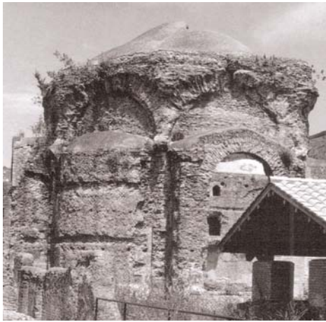
Fig. 2-33: Hadrian's Villa, Water Court, Vestibule exterior looking east, Tivoli (MacDonald and Pinto 1995, Figure 116)
