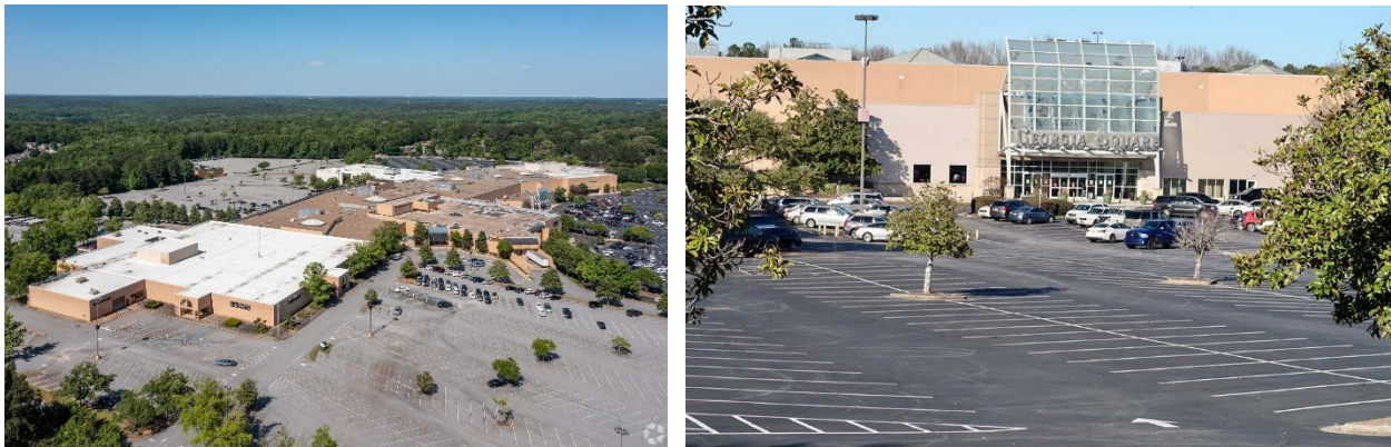
Figure 44: Existing Site Photographs (Source: Peters 2023)
