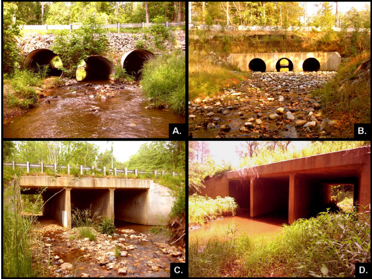
Fig. 2.3. Examples of multiple-barrel pipe and multiple-barrel box culverts from study sites. A.) Canton Creek (Site 1) B.) Unnamed trib to Westbrook Creek (Site 11) C.) Scotts Mill Creek (Site 3) D.) Bluff Creek (Site 6).
