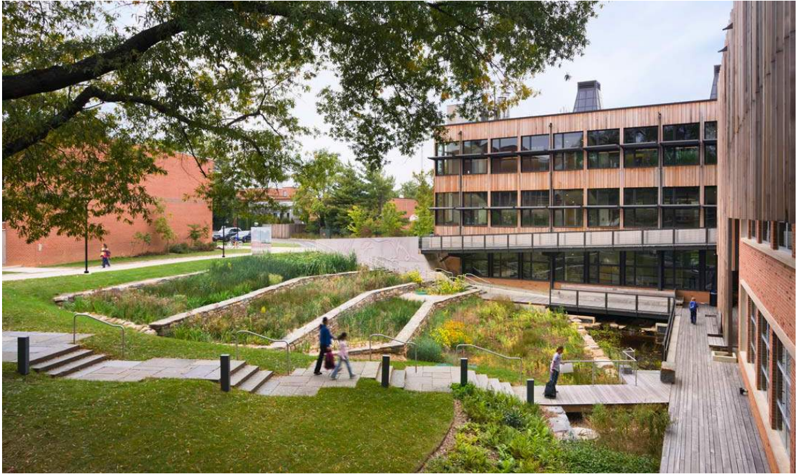
Figure 28. Constructed Wetland and Stormwater Pond (Kieran Timberlake 2015)
