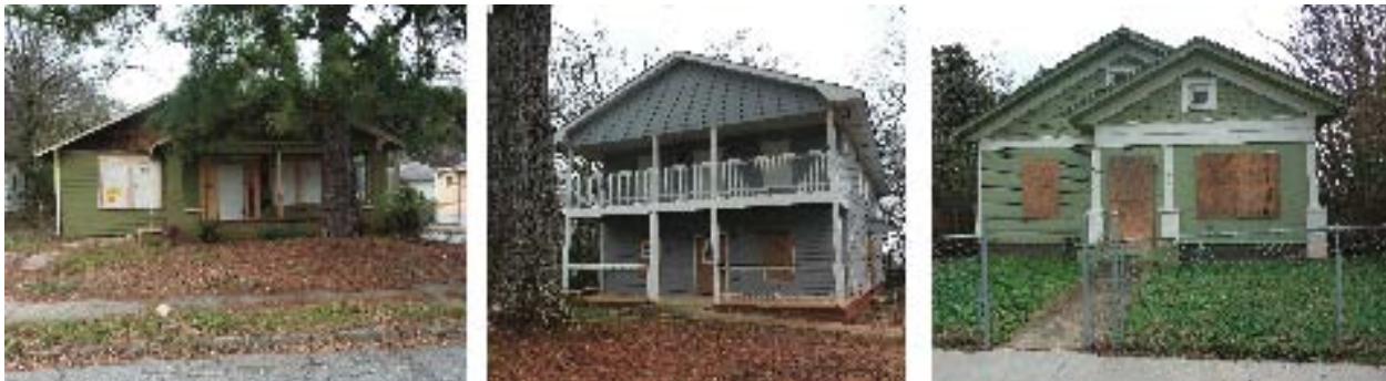
Figure 5. 1 Vacant, boarded-up houses in Pittsburgh (Landers, 2012•)
