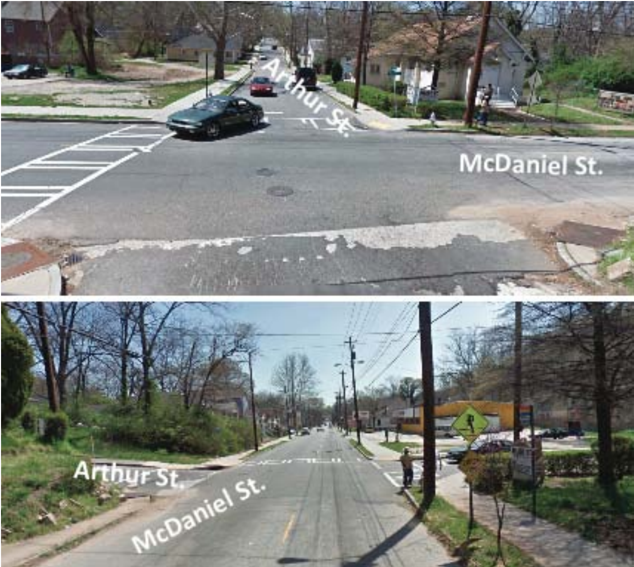
Figure 5. 29 Arthur St. and McDaniel St. intersection, Top: looking West, Bottom: looking South (Landers, 2012...)
