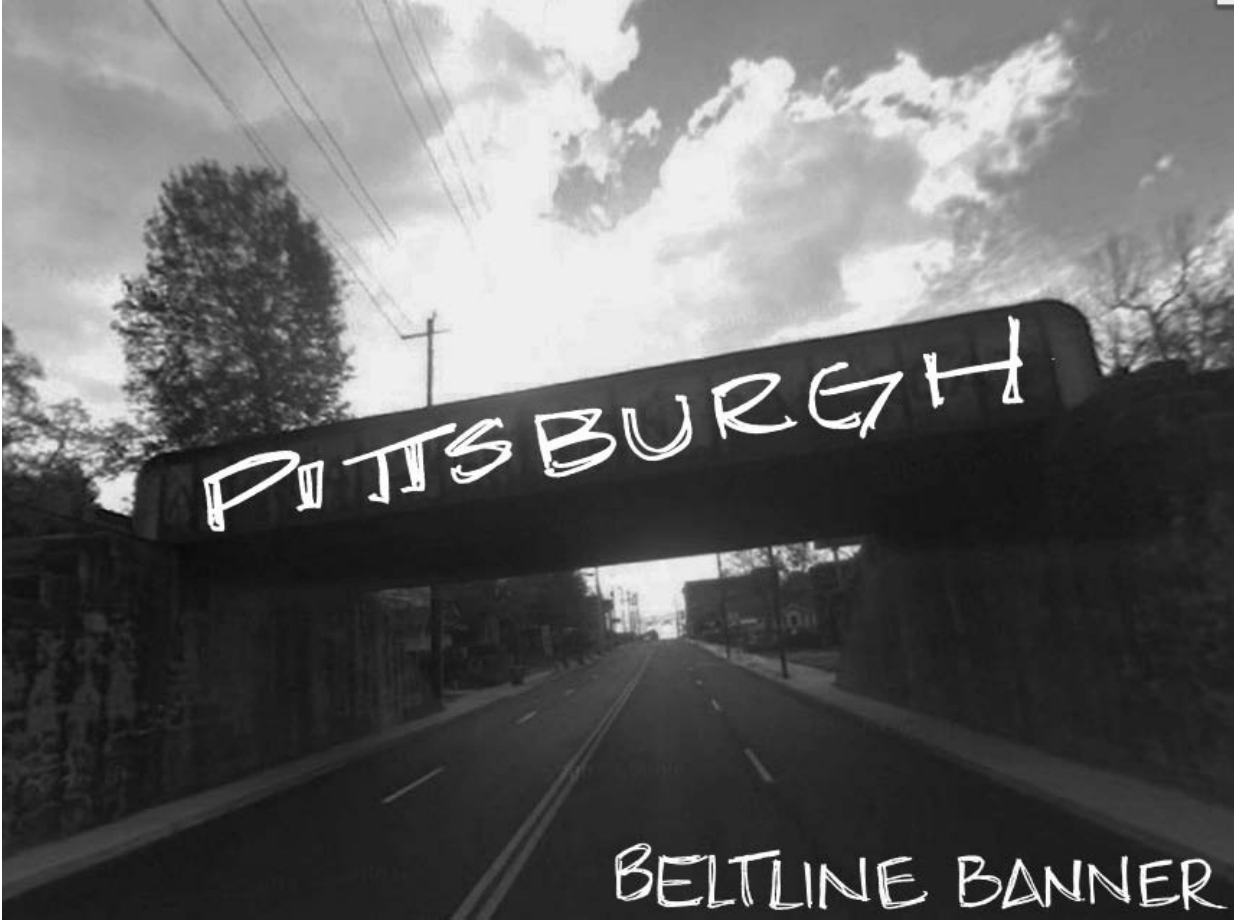
Figure 5. 14 BeltLine overpass heading North, into Pittsburgh (Landers, 2012f)
