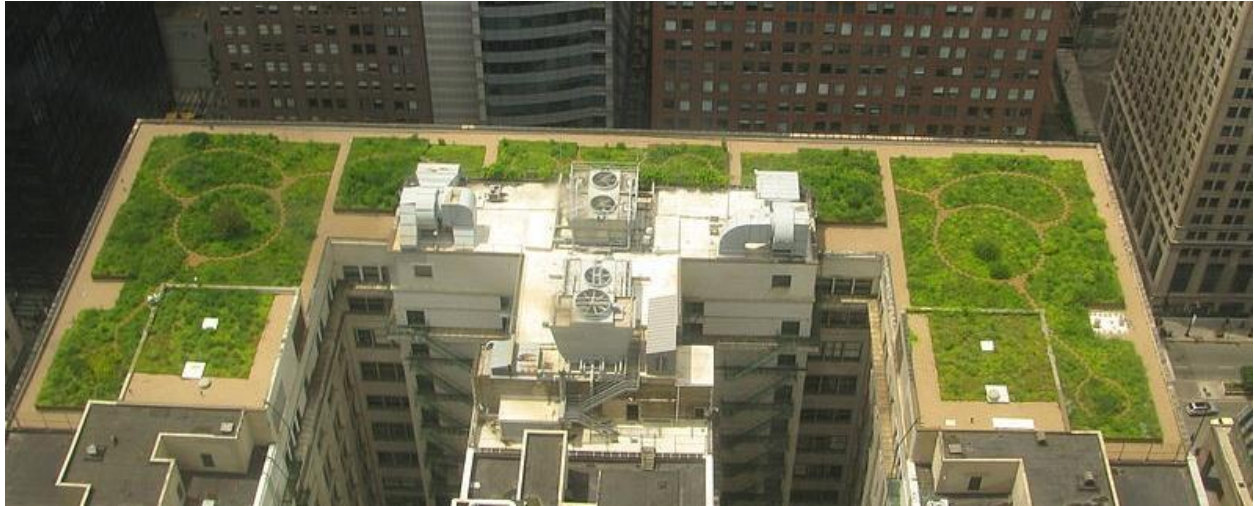
Figure 3.2 Intensive Green Roof over the Chicago City Hall (Ref: www. en.wikipedia.org )
