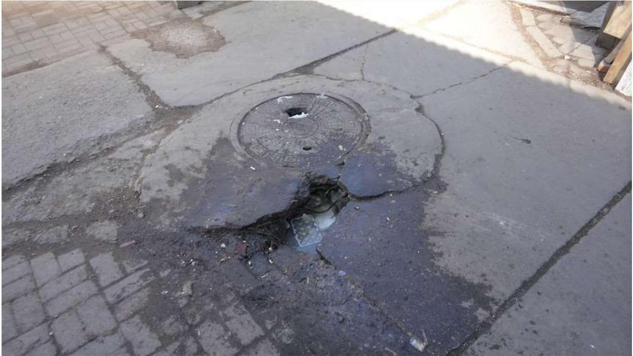
Figure 46. Wastewater gathered in broken pavement
