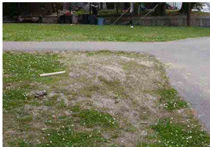
Figure 3.43: Erosion from vehicles turning the corner
