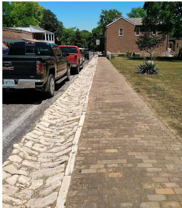
Figure 3.8 Original stones speculated to have been put in place by slaves in Arrow Rock as drains for the main street.
