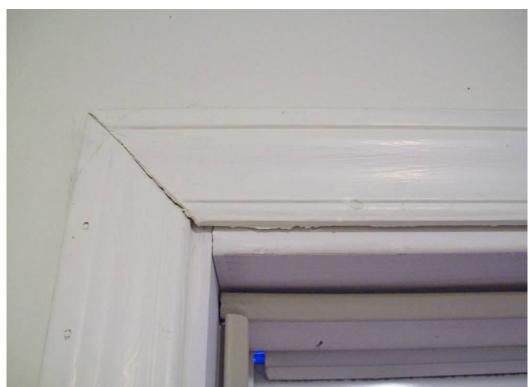
Figure 73: 105 Sammy's Road, Deteriorating Door Frame & Broken Seal, Clearview, Alleghany County, VA (Leonard, 2014)
