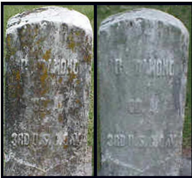
Gravestone before and after pressurized water cleaning
