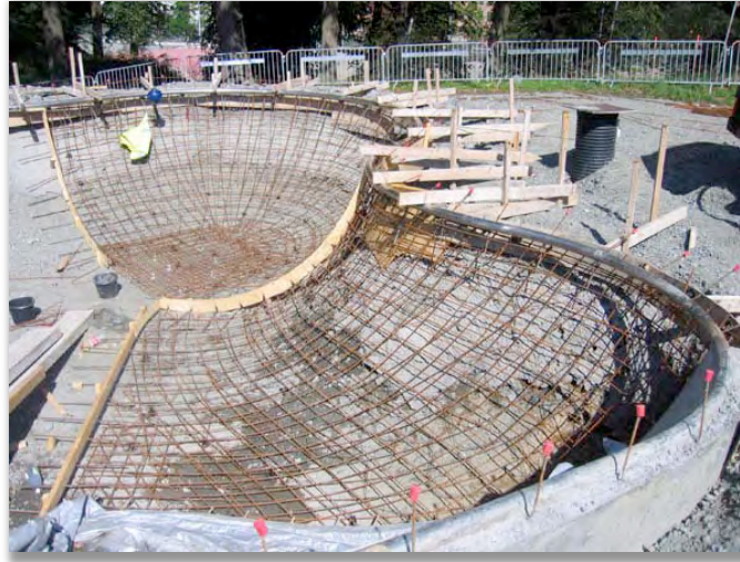
Figure 4.10: Rebar Grid for Concrete Reinforcement
