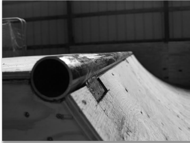
Figure 4.6: Steel Tubing Coping on a Wooden Ramp
