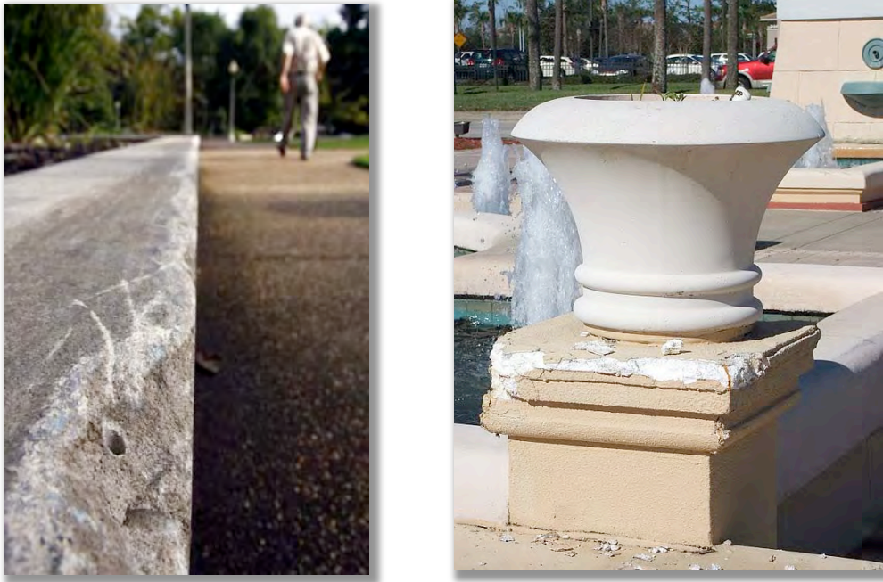
Figure 3.3: Structural Damage Caused by Skateboarding
