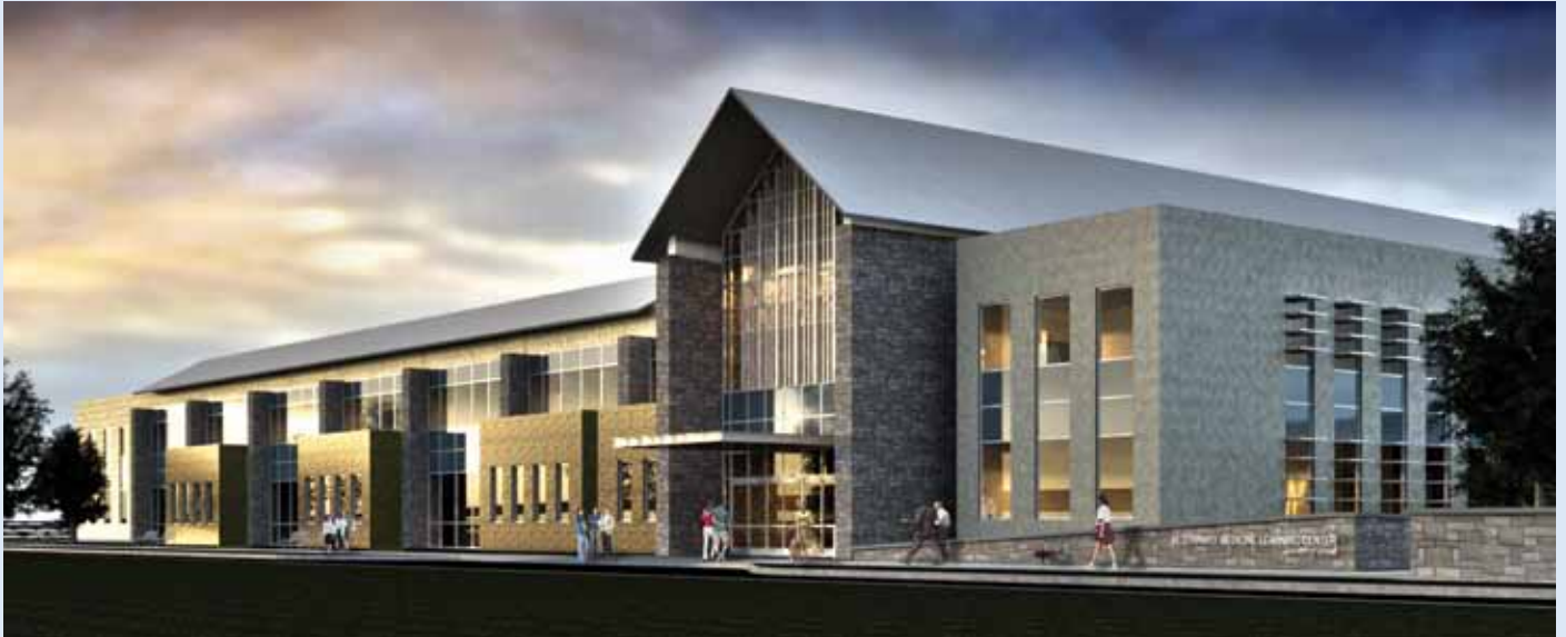
The north façade of the UGA Veterinary Medical Learning Center, facing Southeast.
