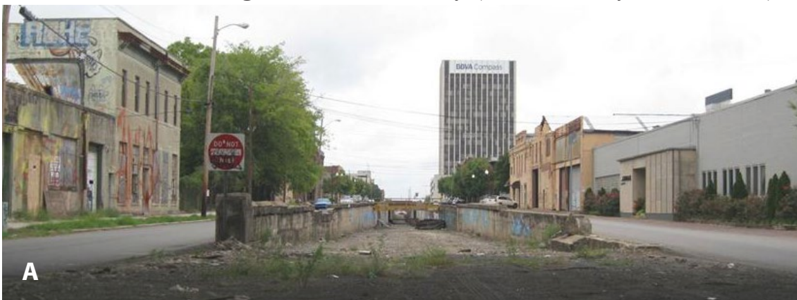
Figure 5.2: Pre-construction photos of the “First Avenue Cut,” walking west from 24th Street. Letters relate to Figure 5.3: Site Inventory. (Photos Courtesy of Jason Crunk)
