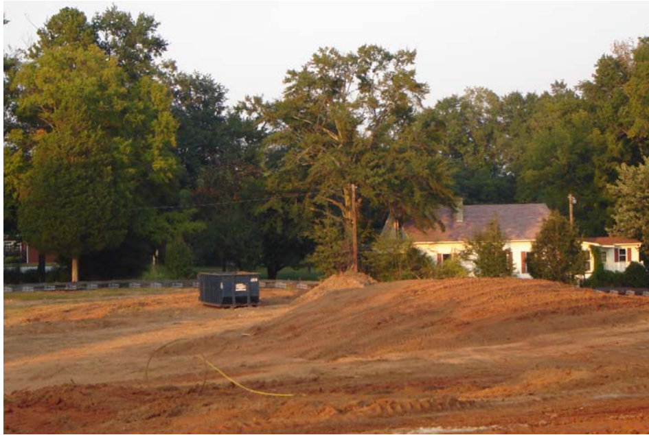
Figure 2.8: Bulldozers remove all reference to the natural lay of the land. Here a slope and all vegetation are being removed to create parking for the new strip mall.
