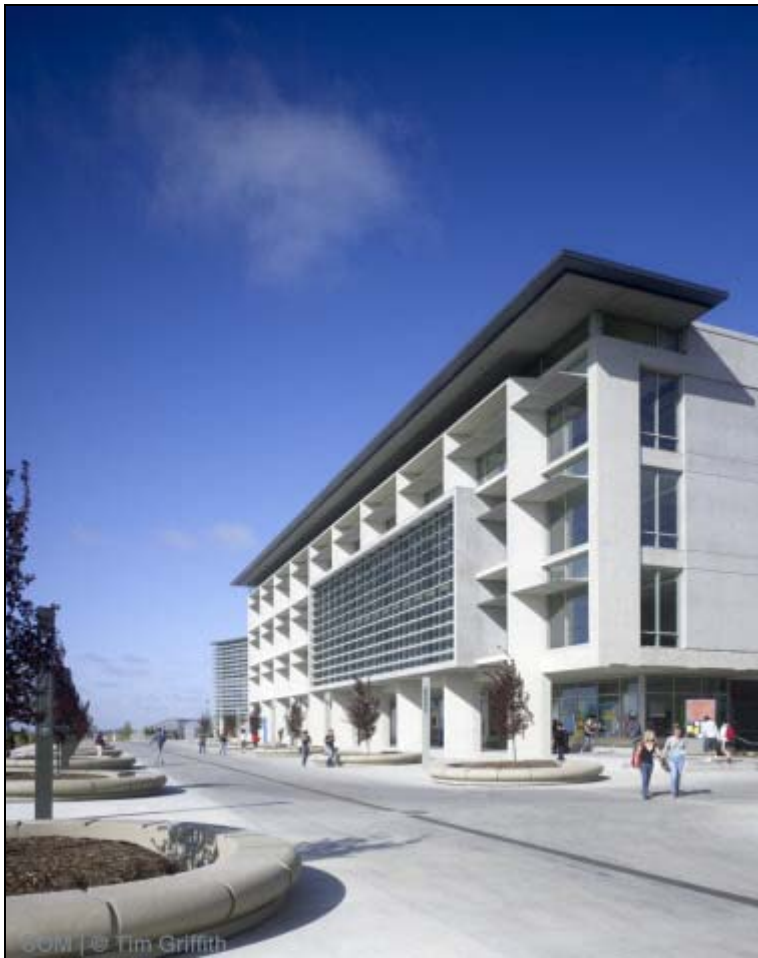
Figure 7.3: Library at University of California at Merced – Sun Shading Devices
