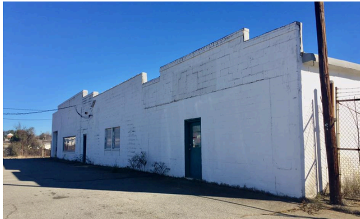
Figure 69: West elevation of the Tru-Ade Bottling facility, which features two block-glass windows, a strip window, a glass-front loading bay, and two entrances. The building was built of concrete block and features a stepped sign board. Due to the busy state highway in front of this building, I was unable to get a direct elevation photograph (Author.)
