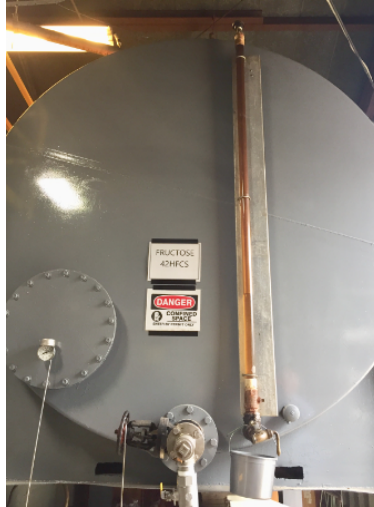
Figure 41: Original tank used to hold additional ammonia, now repurposed to hold fructose corn syrup for candy making (Author.)
