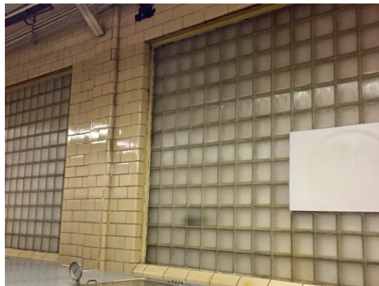
Figure 46: Original glass block windows in the south portion of the factory, dating to 1948. They have been covered from the outside for security reasons. The cream-colored tile is also original to 1948, as indicated in the June 19, 1949 Macon Telegraph (Author.)
