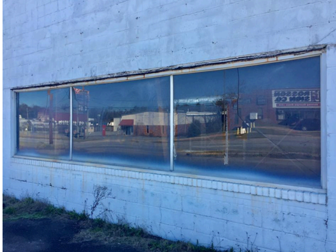
Figure 74: Strip window on the west elevation of the Tru-Ade Bottling facility. Like the glass-block windows on the same elevation, this strip window was framed in brick. The original iron frame is still visible around the strip windows, as evidenced by rust and iron jacking. A crack is visible in the bottom right corner, traveling through the concrete block towards the ground. Vegetation presents the problem of rising damp. Water could potentially be entering the building from the window frame (Author.)
