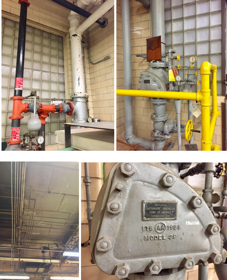
Figures 49, 50, 51 & 52: Original sprinkler system for fire suppression, currently not in use (Author.)
