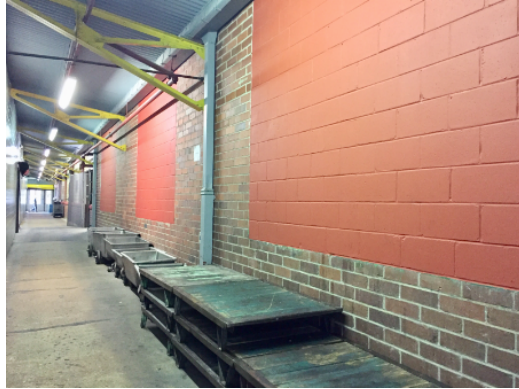
Figure 33: Original east elevation, which is now enclosed to form a corridor. This was the original exterior of the 1948 building. The original concrete floor was the loading dock, and the original exterior brick wall (now interior) is visible. Original windows were removed and filled with concrete block, which damages some of the integrity of the structure, but was necessary for safety reasons (Author.)
