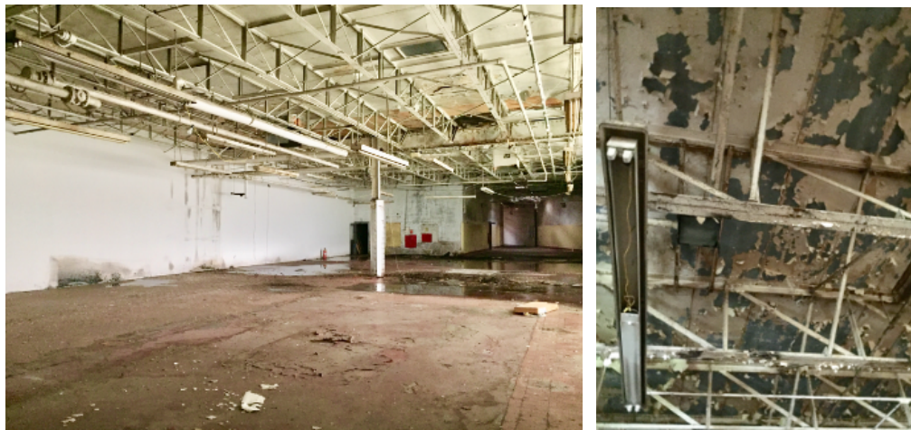
Figures 62 & 63: Interior of the south elevation, facing east showing water damage. Water damage is visible along the wall, coming from the roof (Author.)
