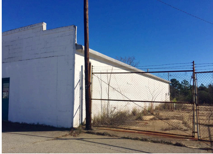
Figure 70: South elevation from the southwest corner of the Tru-Ade Bottling Facility. The building features a small overhang at the roofline. This photograph shows that the stepped cornice on the front is a parapet and sign board. Exterior problems include vegetation growing along the outside of the building, mostly grasses, weeds, and vines, but at least two potential trees. If allowed to grow, these could affect the foundation. Grasses and weeds create the potential for rising damp (Author.)
