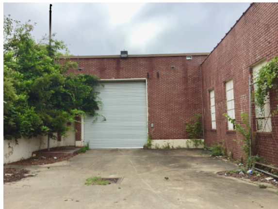
Figure 59: A portion of the west elevation, featuring a recessed loading bay. The windows face north. The window frames are original to the structure, though the glass is missing. This elevation shows ample vegetation growing around the building. Some salt efflorescence problems are visible on the north-facing brick wall between the windows (Author.)
