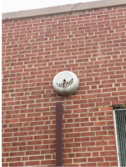
Figure 56: Exterior alarm dating to the mid-twentieth century. Strip windows are visible in the lower right portion of the photograph. Evidence of water damage is visible along the top of the window beneath the brick, and as evidenced by the structural cracks moving upward from the corner of the window towards the roof of the structure, through the bricks and mortar (Author.)
