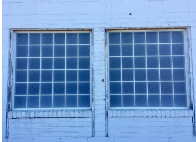
Figure 72: Glass block windows on the west elevation of the Tru-Ade Building. Popular in the mid-century, these frosted glass blocks are set thirty-six to a frame. Wooden boards were added to the sides for stabilization, but the original iron frame is still located at the top of the windows. The windows were originally faced in brick instead of concrete block (Author.)
