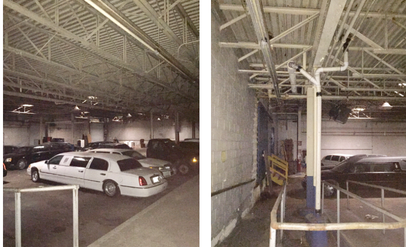
Figures 64 & 65: The west interior is currently used to store funeral vehicles for the funeral home. This portion of the facility is in less disrepair than the south portion. The roof has been repaired and the trusses do not show signs of flaking paint. The concrete floor is clear of debris. Originally, this area was of the production line for Colonial Bread. The only current electricity is within this section of the building (Author.)
