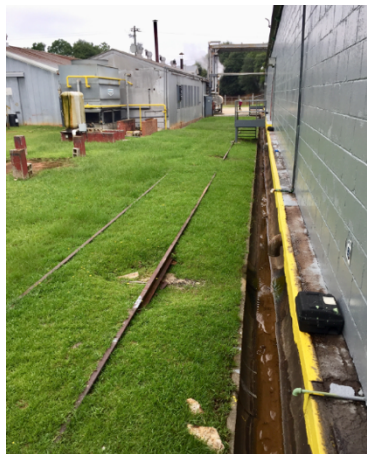
Figure 32: East elevation, looking south. This photograph shows the original railroad line spur, which ran north to south, parallel to the east loading dock. The gray concrete wall is a modern addition to enclose the loading dock and create an interior corridor (Author.)
