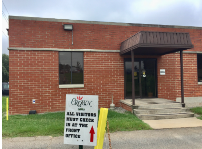
Figure 30: North elevation of the addition, built in the 1970's. The brick color tone is darker than the original brick. The front stoop and porch roof were added at the same time as the addition. The upper stringcourse was carried through from the original building to make the addition appear continuous (Author.)
