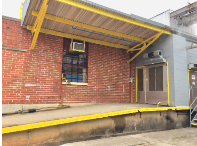
Figure 31: The original 1948 northeast elevation from the exterior. The 1970's corridor addition (which enclosed the loading dock) is constructed of concrete block painted gray. The original loading dock is visible, sloping downward. The windows are also original (Author.)
