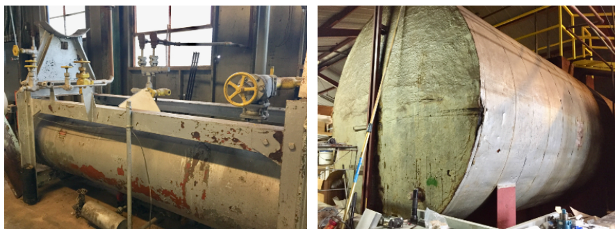
Figures 39 & 40: Original ammonia tanks, located within the secondary structures. The second tank has been repurposed to hold diesel fuel (Author.)
