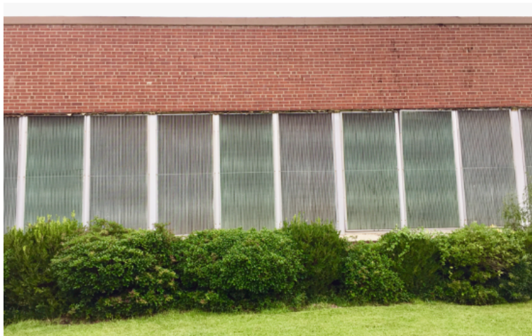
Figure 57: Mid-century strip windows along the south elevation of the structure. Water damage is visible at the top of the windows, just below the brick. Some windows are also loose from their frames allowing water to enter the building, as evidenced by the second window from the right (Author.)
