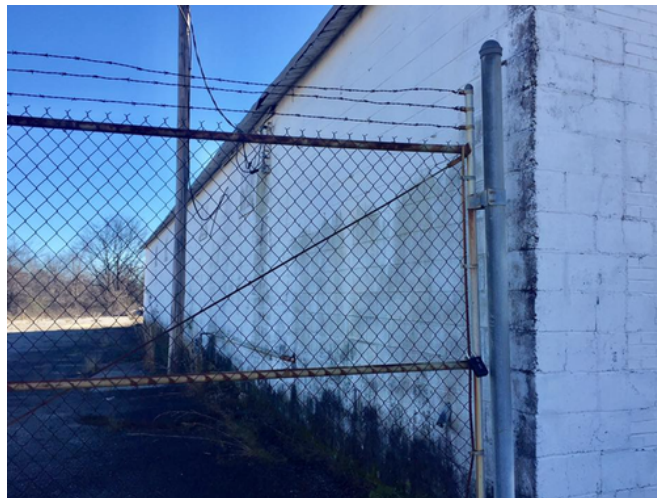
Figure 71: North elevation of the Tru-Ade Bottling facility. This elevation shows problems with rising damp, stemming from vegetation and moss growing along the bottom of the structure. Though the building has been painted, rising damp causes problems by attacking mortar (Author.)
