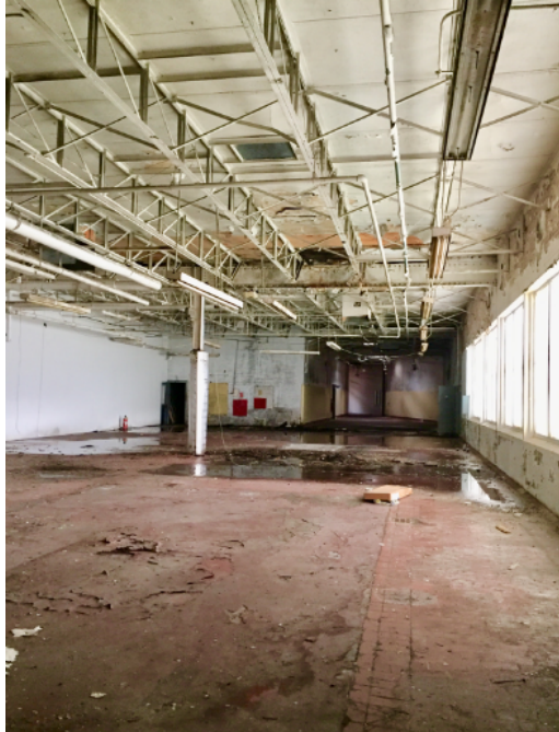
Figure 61: Interior of the south elevation, facing east. This room was once part of the bread production line. Water damage is clearly visible by the large puddle in the center of the space. It appears water is entering the building from the roof and windows (Author.)
