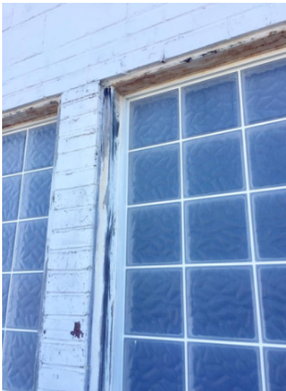
Figure 73: Detail of glass-block windows on the west elevation of the Tru-Ade Bottling facility showing the wooden boards added to the sides of the windows. The tops are still iron, evidenced by the rust. The windows were originally framed in brick instead of concrete block. The same types of glass blocks were also used in the Durkee Factory, built in 1948, and are present in another bottling facility located across the street from the Tru-Ade facility (Author.)
