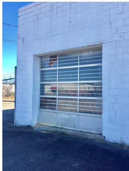
Figure 75: The loading bay on the west elevation originally allowed trucks to load and unload product. The windows were added at a later date (Author.)
