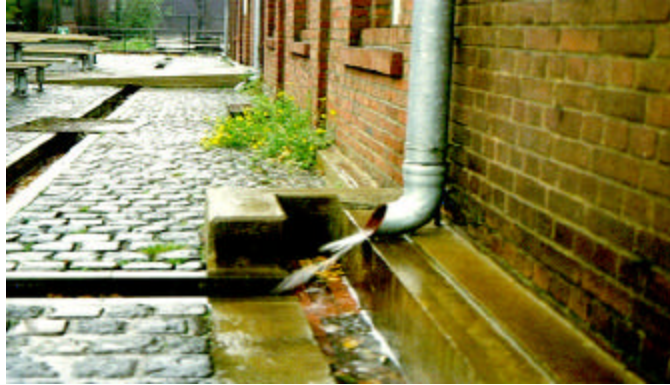
Figure 2.1 – Stormwater drainage runnels
