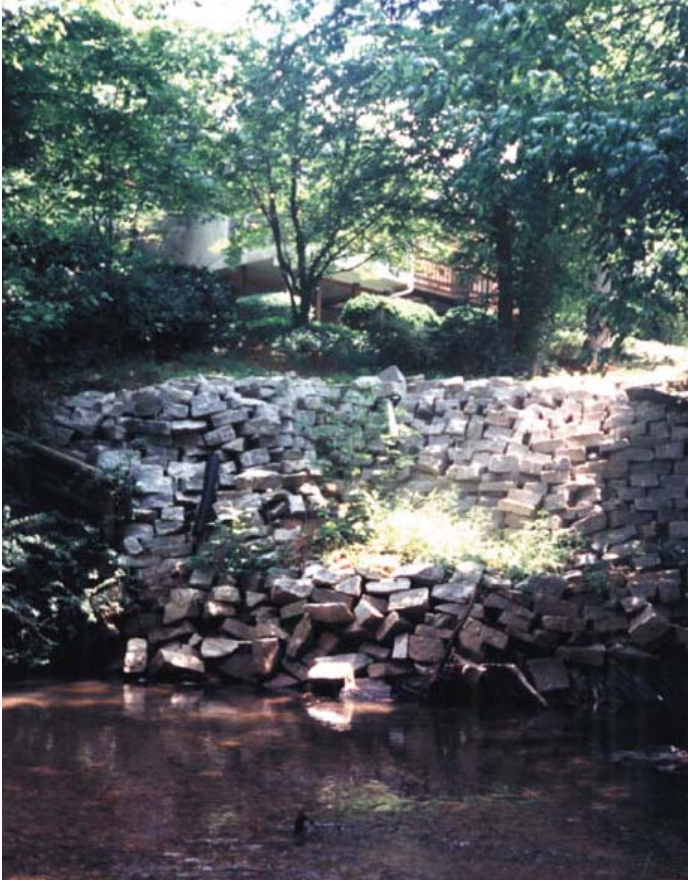
Figure A.2. Photographs of Unrestored Site, Nancy Creek at Murphey Candler Park, DeKalb County, GA. a)severe bank erosion, b)rip-rap and baseball fields on right bank, c)little riparian vegetation and failed bank stabilization on left bank.
